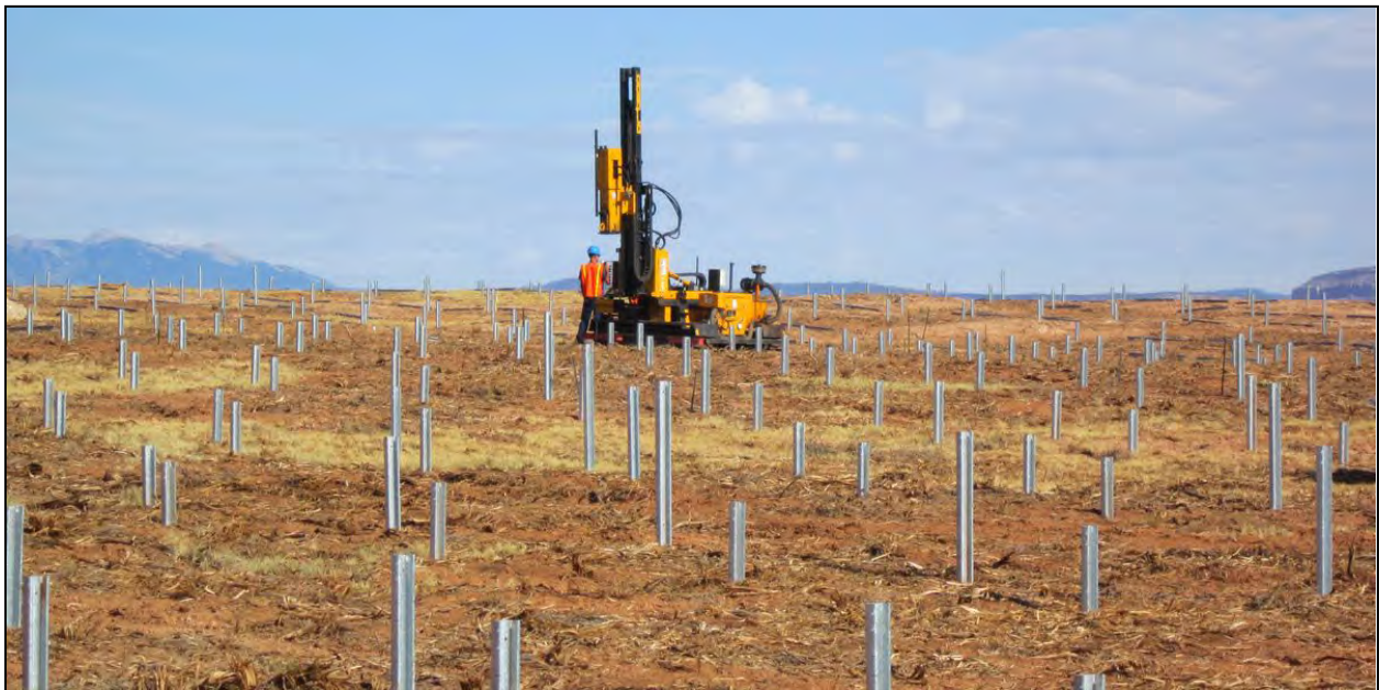
Inset 1. Typical steel support beams for PV panels and pile-driver during construction. (Photo credit: Clean Energy Collective).
