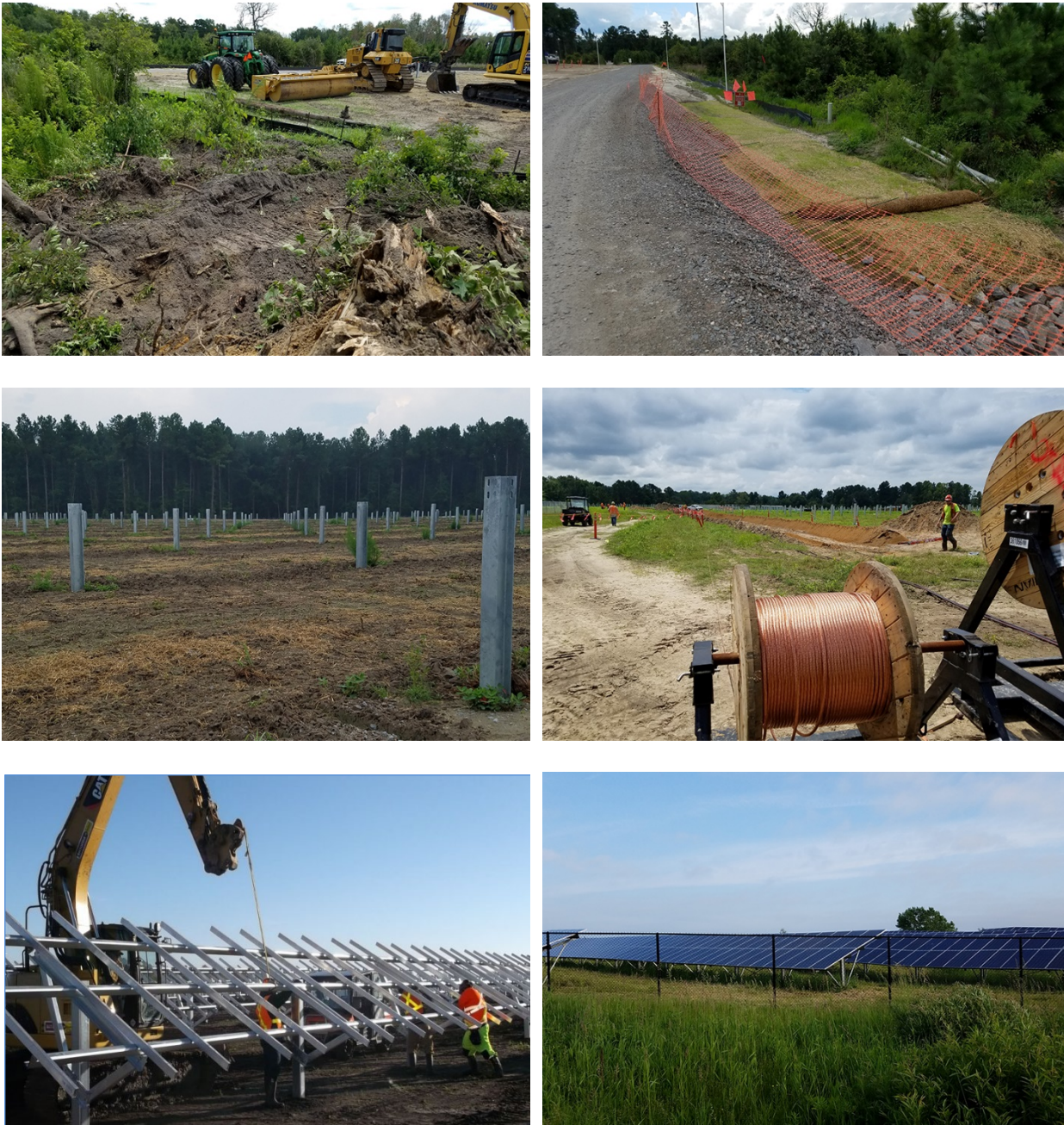
Figure 5.3-1 Representative Photographs of a solar facility during construction.
